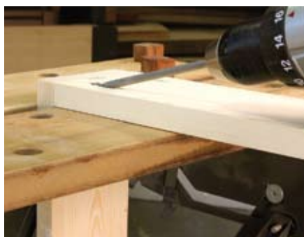
Building the drawer with pocket screws is a simple task. But, it is necessary to achieve a flush fit between the front and sides. The level joint makes the best connection when attaching the drawer face with glue.
