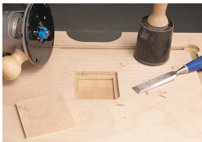
After cutting the hole with a jigsaw, the opening is rabbeted using a bearing-piloted router bit. Then chisel the corners square and fit the replaceable insert plates tightly into the rabbet. Make a couple extra insert plates.
