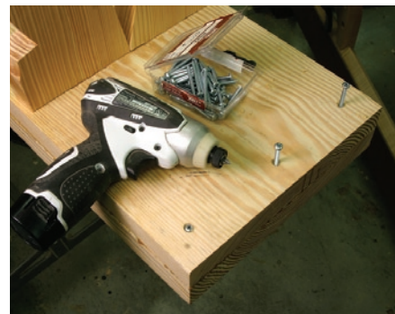
Cheap clamps. With the seat planks glued together, drive 2" screws through the underside to clamp things up. Place a screw wherever you see a gap between the planks.
