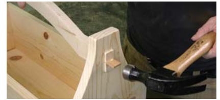
Wedgie. After using a handsaw to cut a kerf in the center of each end of the handle, paint your wedges with glue and tap them in. After the glue dries, trim the wedge flush with the end of the handle.
