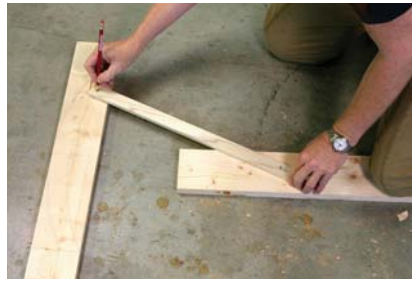
Scrap trammel. It's simple to make a trammel to lay out large curves. Drill a pencil hole at one end of a flat, straight piece of scrap. Measure the distance of the diameter of the required circle (in this case, 16"), and use a nail to secure the other end of the stick to a piece of scrap the same thickness as your workpiece. Line up the trammel on the centerline of your workpiece, then mark the curve.
