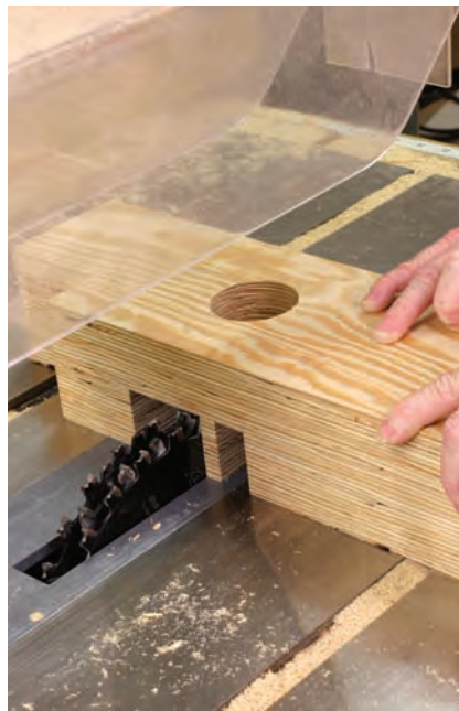
Right wasted. Use your dado-stack set-up to remove the waste for the threaded nut block. Be careful to work right up to the lines and test the fit of the block into the dado.
