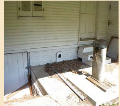
No spring. Unlike a spring house that would have water running through it, the Milk House at White Water has a pump outside that directed water through a pipe into troughs inside. Presumably, cool water was pumped into the structure by passers-by.
